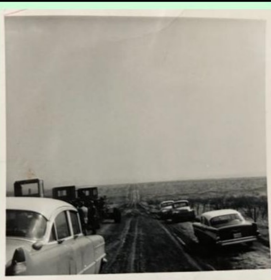
Pictured: Cutting the dirt road to Roaring Springs Camp in 1962.
